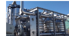
Zeolite adsorption + catalytic oxidation furnace (CTO)
