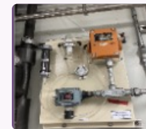
The nitrogen system keeps the oxygen content < 5 vol%
